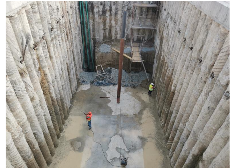
3 rd PRIZE: Cleaning of Piles
