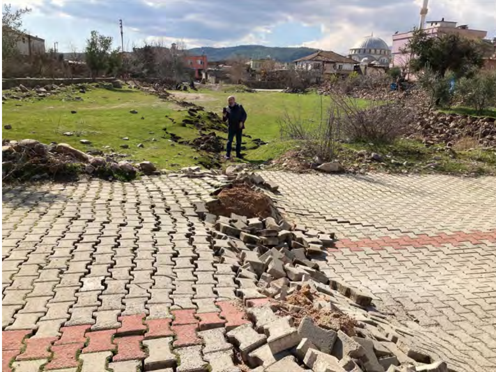
Figure 17: Surface rupture observed in residential neighborhood near Hessa (Source: https://twitter.com/ziyadin/status/1623288689894871046/photo/1 )
