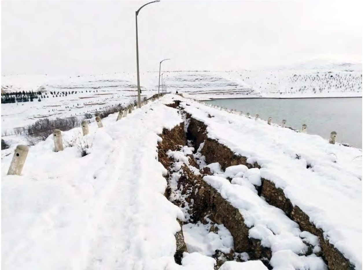
Figure 29: Cracking damage observed in the Sultansuyu Dam (Source: https://www.ntv.com.tr/galeri/turkiye/govde-aksinda-catlaklar-olusan-malatyadaki-sultansuyu-baraji-tahliye-ediliyor,xxRN92Huy0iiG0tyCNU4fA/aimTJcX5X0egL7OUo5ez0Q )
