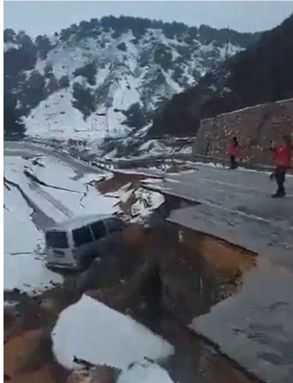
Figure 22: Lateral flow landslide on the road between Adana and Gaziantep (Source: Twitter video Sokagin Sesi Gazetesi; https://twitter.com/sokaginsesigaz1/status/1622689001332215853 )
