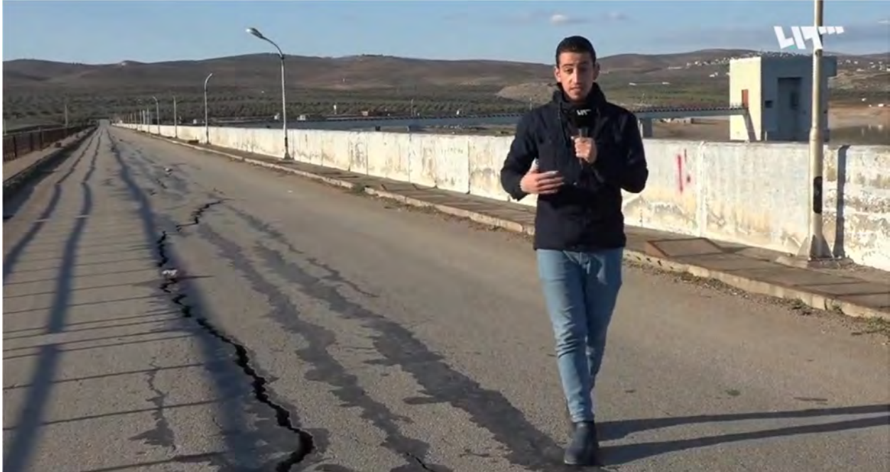
Figure 27: Cracking in the Afrin Dam (Source: https://twitter.com/Hibakarm/status/1623723294686838784 )
