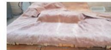
Fig.10: 24h curing with wet burlap
