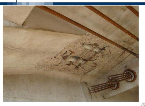
Damage observed on the precast element during the tensioning phase
